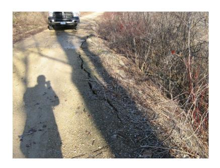
Slope showing stabilization problems
