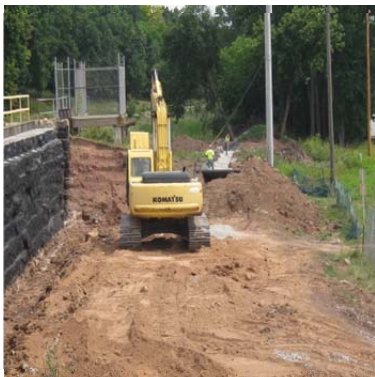
RH chamber wall backfill under way Lock # 1
