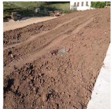
Lock #1- LH backfill to rough grade
