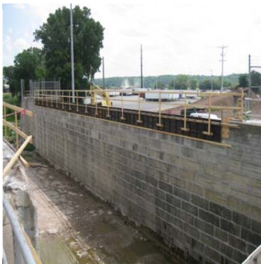
Lock #1-RH formwork for sidewalk
