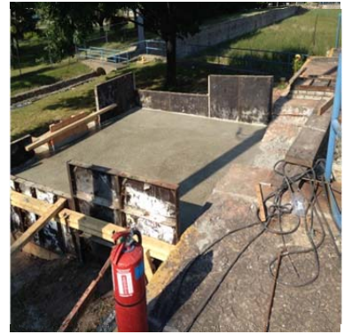
Lock #1- LH downstream spar/tripod slab foundation
