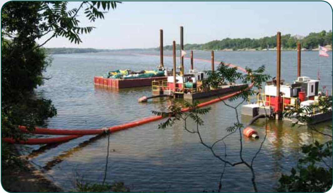
There are two PCB removal practices at work in the Lower Fox River. Either the PCBs are sucked off the river bottom by a dredge, then taken to a toxic waste landfill ( right ), or sand and gravel is dumped on them, essentially burying them ( above ). The sand and gravel operation took place on Little Lake Butte des Morts, at Menasha. The dredging operation happened just downstream of the dam at De Pere. (Photos courtesy Wisconsin Dept. of Natural Resources)
