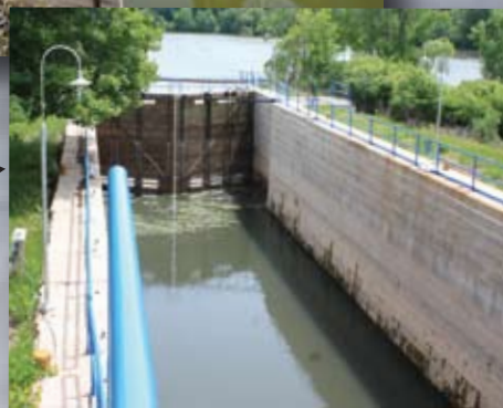
Combined ▶ Locks Lower Gate and Restored Walls June 2009
